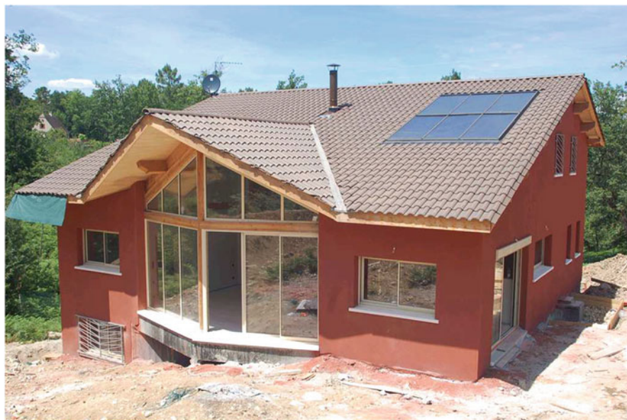
Fig. 6.1 View of the south façade of a 2-floor single-detached house located in south west of France. (From Moujalled et al. 2018). The walls are made of 30-cm thick coated sprayed hemp-lime concrete supported by a timber frame structure
