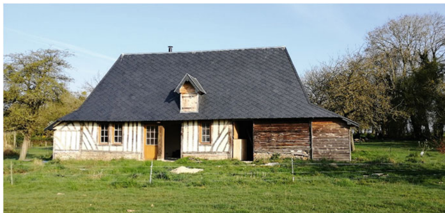
Fig. 2.7 A half-timbered building in Normandie, France, dating from the early nineteenth century. The walls and slabs were renovated using different solutions based on hemp concrete. (Source: with the kind courtesy of Florence Collet (Rennes, France) and Yacine Aït Oumeziane (Belfort, France))
