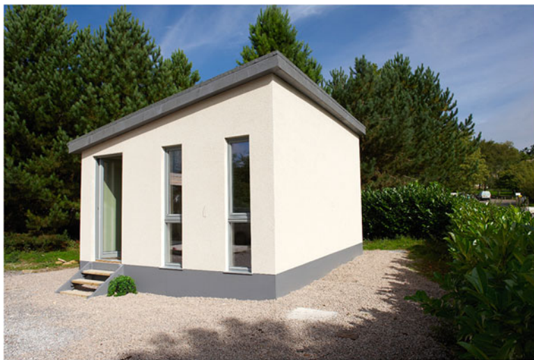
Fig. 6.13 View of the instrumented hemp concrete building 'Hempod' in Bath, England (Shea et al. 2012) © Mike Lawrence, University of Bath
