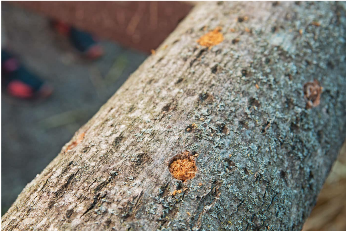
Drilled holes filled before sealing
