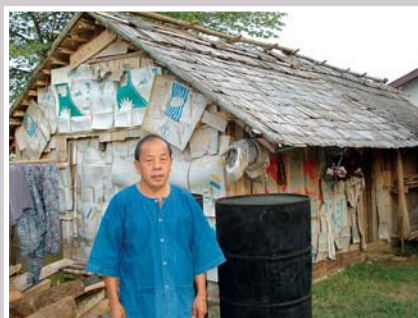
Figure 26. Corrugated paper from old boxes is used for the walls and ceiling. These carton box materials are already over 3 years
