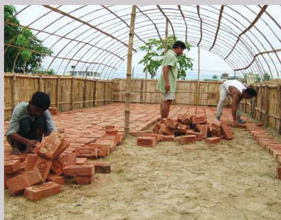
Figure 5. Floor work for growing house
