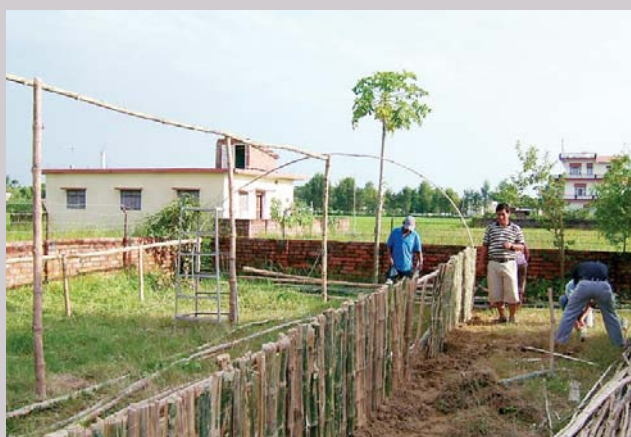
Figure 4. Growing house under construction
