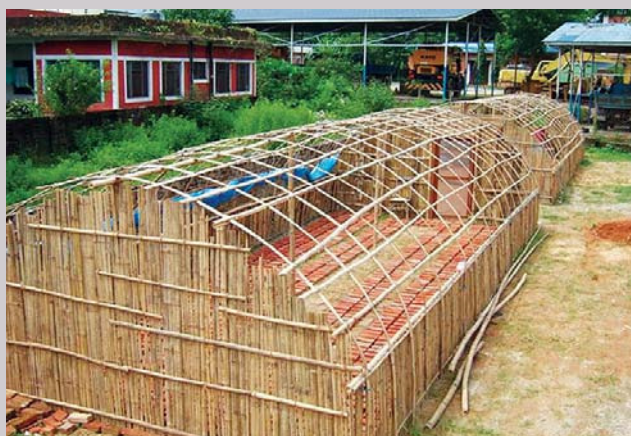
Figure 6. Two plastic tunnels
