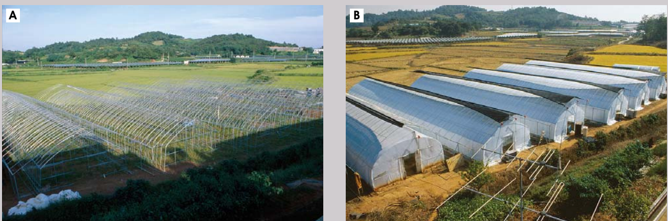
Figure 11. Growing houses with threefold structure under construction A: Completed framework B: Completed covering with plastic films and shading nets
