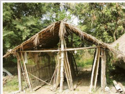
Figure 32. Rack frame structure
