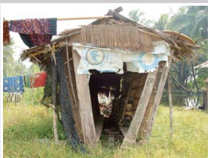
Figure 24. Imperata grass roof with two stacks of substrate bags as the walls
