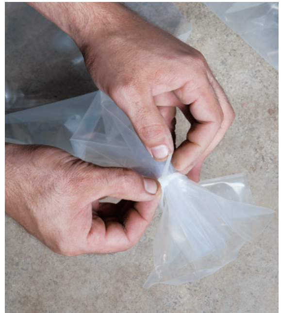
Seal the ends of columns securely with zip ties.
