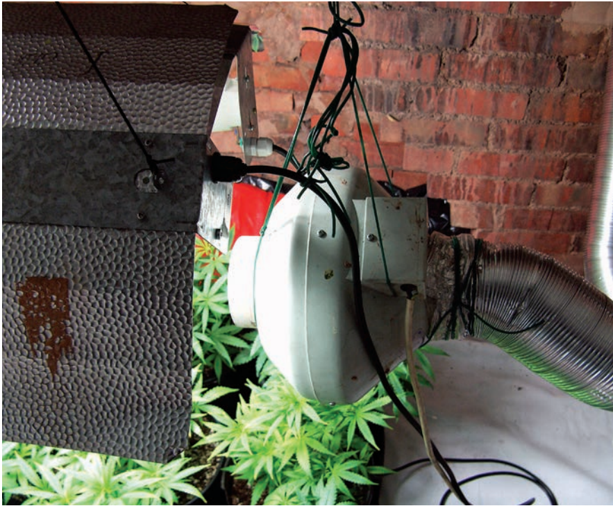
This fan vents directly from the lamp area to remove the excess heat generated by the bulbs.
