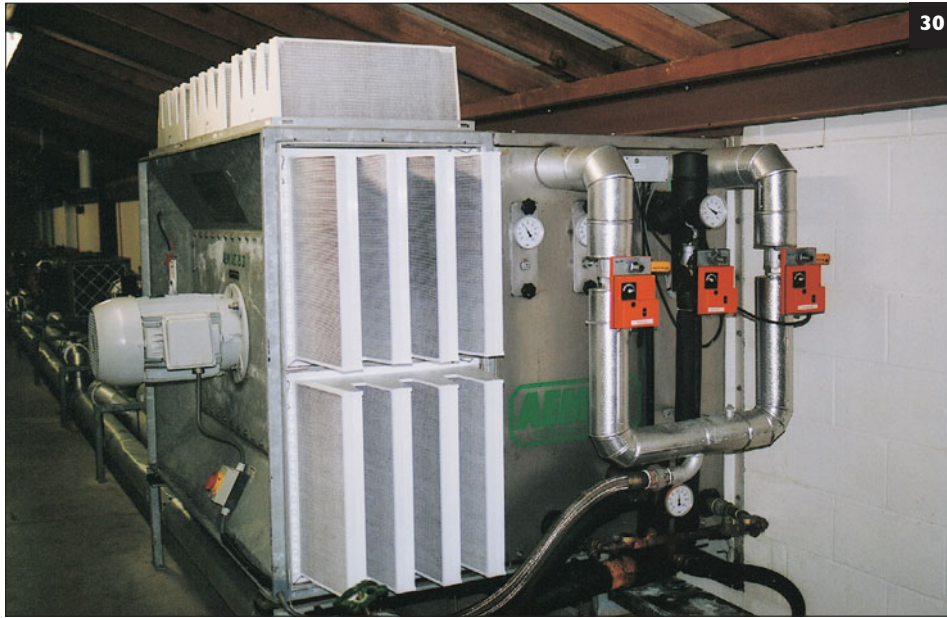
30 A large absolute-filter assembly with the filter units projecting. This assembly is in the roof space above the units requiring filtered air.
