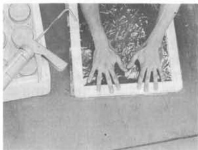
fig. 19: Clear plastic vinyl is glued over the window.
